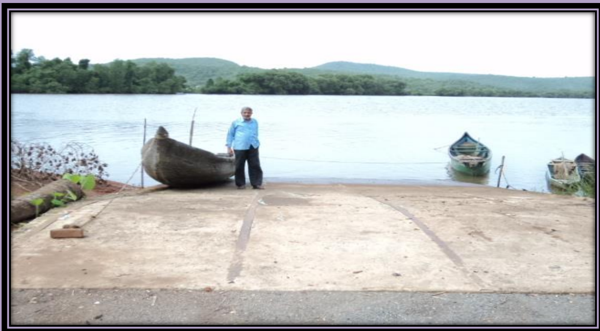
RAMP AT ULLANDO
